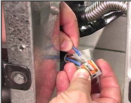
Figure 3: Connecting drain safety wiring.
